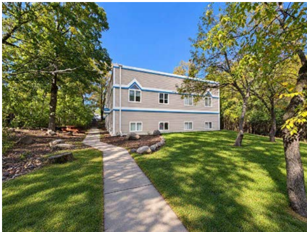
Back Side of Building
