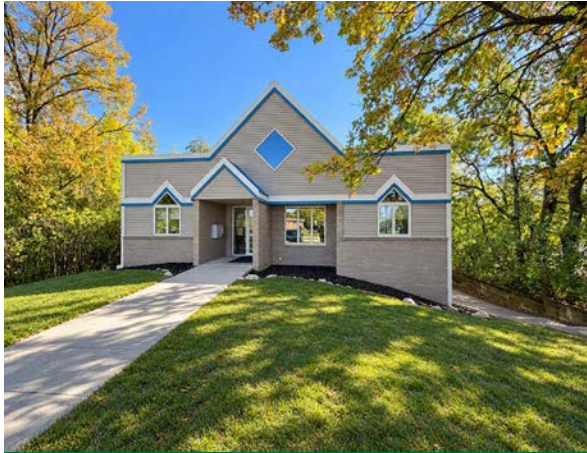
Front Side of Building
