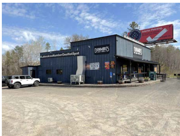
West Side of Building
