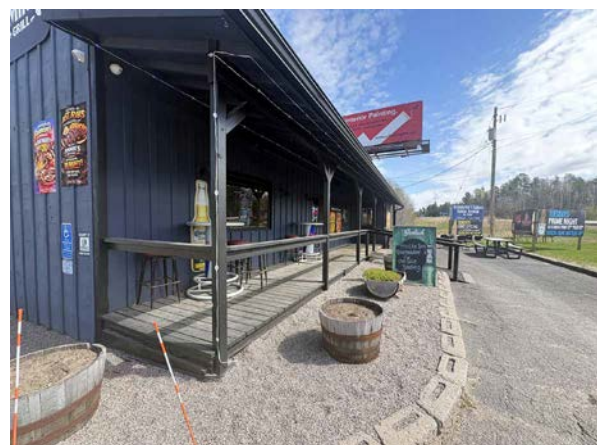
Front Porch & Entrance
