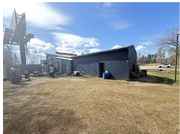
East Side of Building
