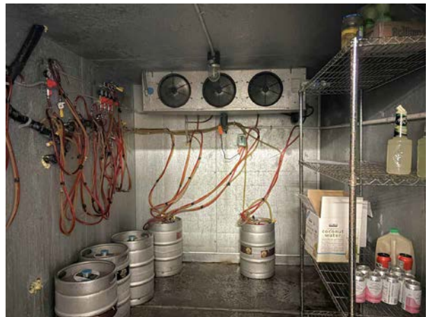
Lower Level - Walk-In Cooler
