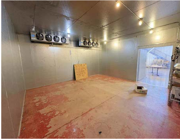
Lower Level - Walk-In Cooler
