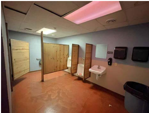
Lower Level - Restroom
