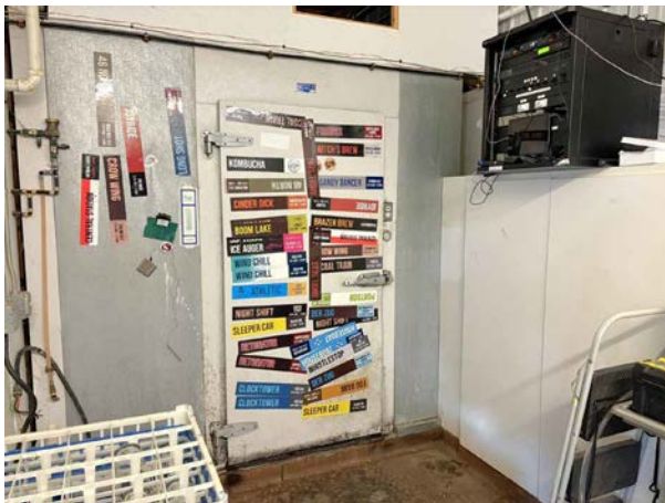
Lower Level - Walk-In Cooler
