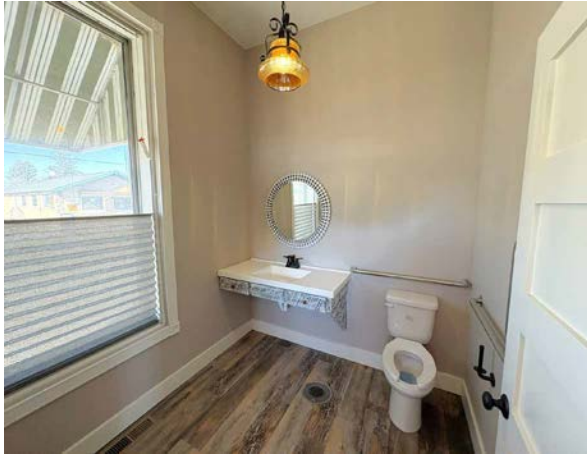
Restroom (ADA Compliant)
