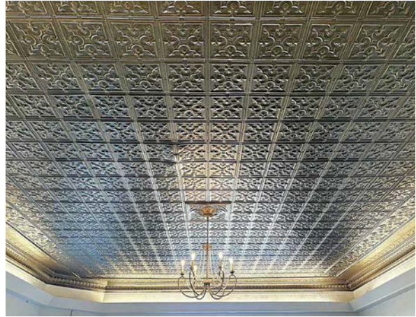
Original Tin Ceiling
