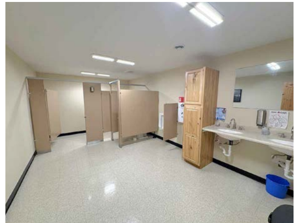
East Office - Restroom
