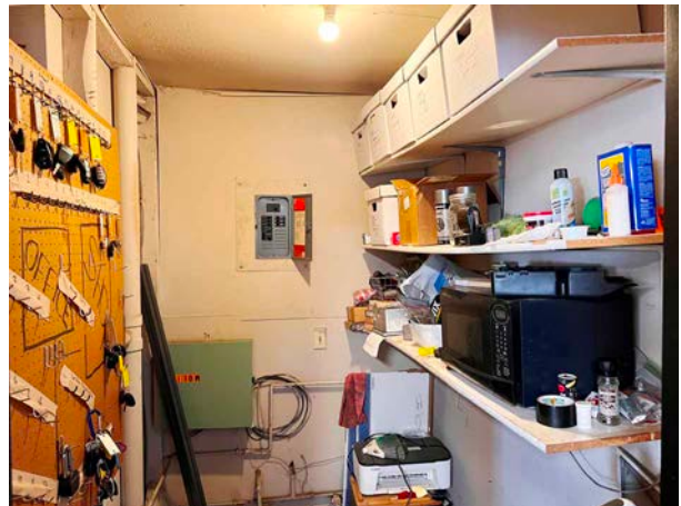
Office Building - Mechanical/Storage Room
