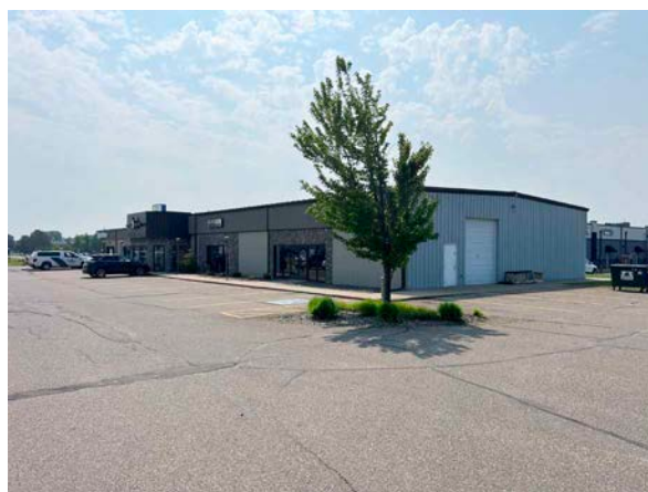
Unit #5 (West Side - OH Door)
