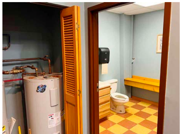
Upper Level - Restroom
