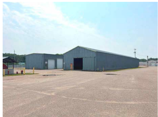
Buildings E & F
