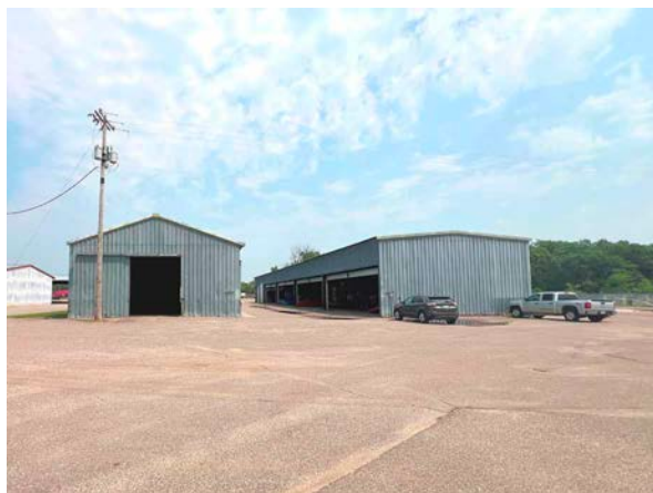
Buildings E & F
