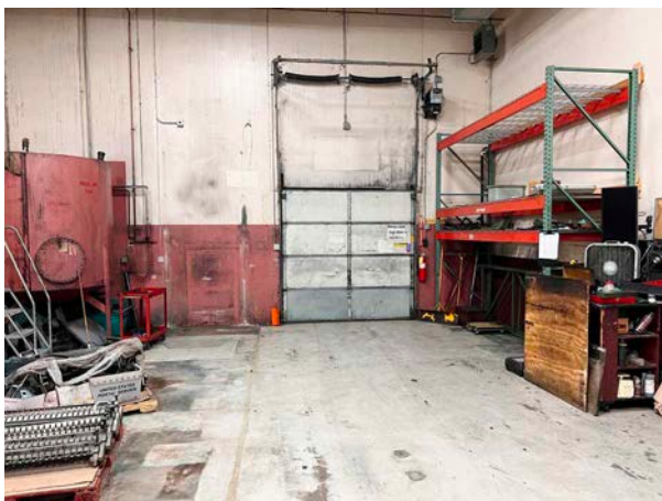
Front Warehouse Drive-In Door
