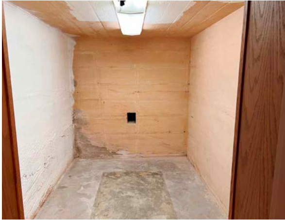
Lower Level - Vault
