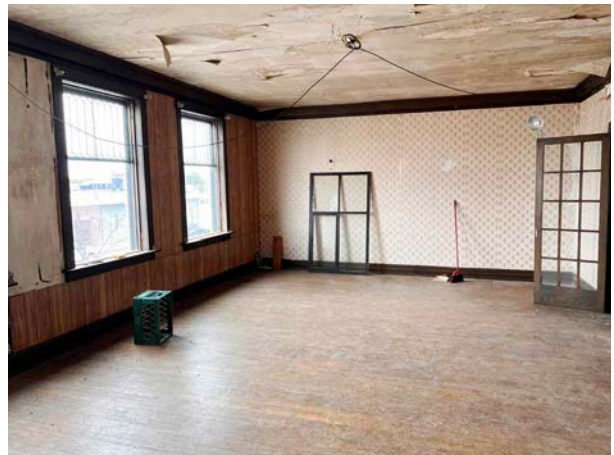
Upper Level - Living Room
