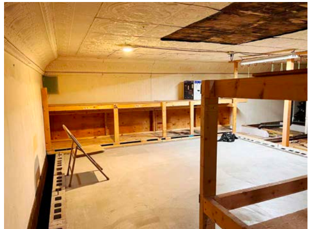
Main Level - Upper Storage
