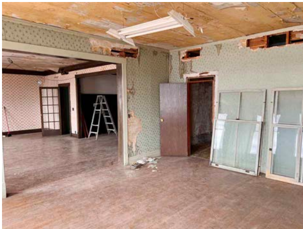
Upper Level - Living Room
