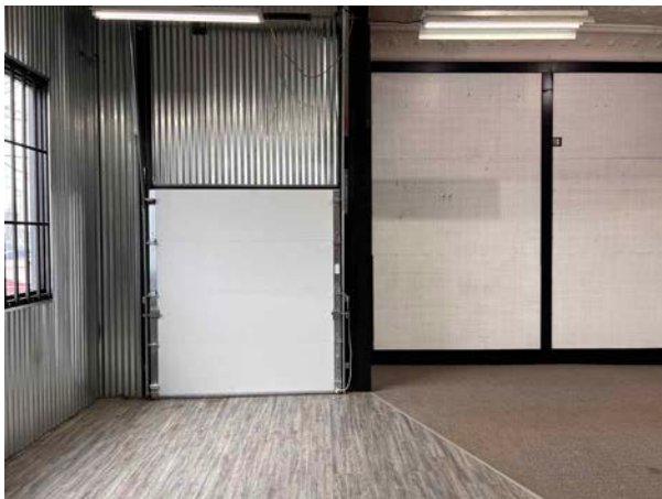
Main Level - Service Door
