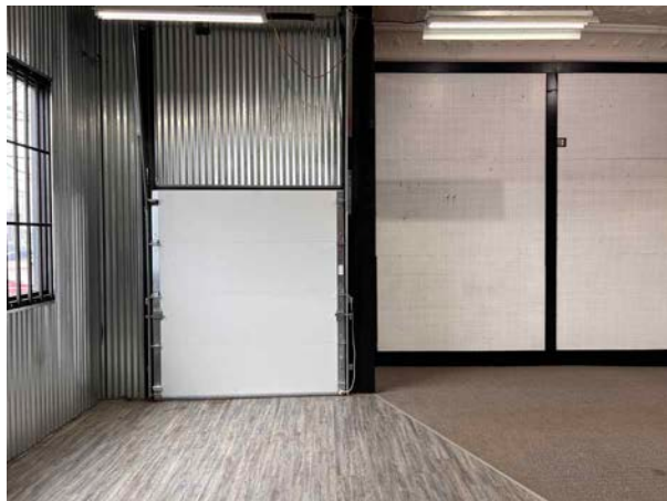
Main Level - Service Door
