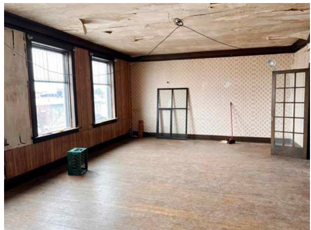
Upper Level - Living Room
