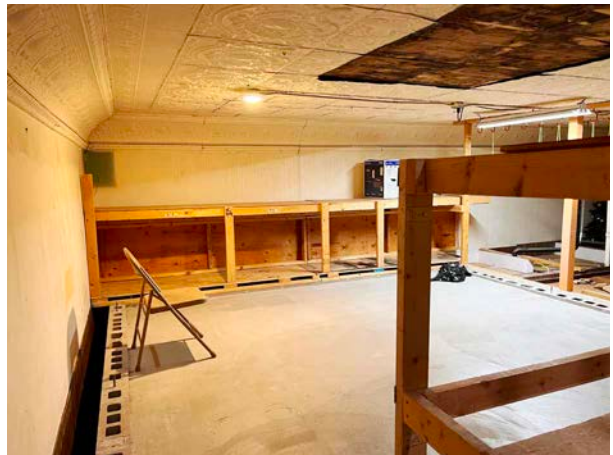
Main Level - Upper Storage
