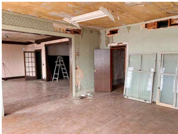
Upper Level - Living Room
