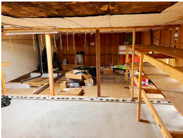
Main Level - Upper Storage
