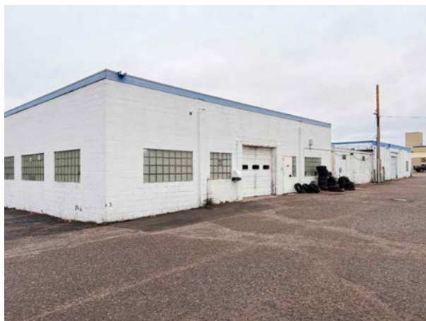
Subject Building - South Side
