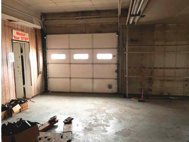
North Drive-In Door Area
