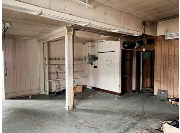
North Drive-In Door Area
