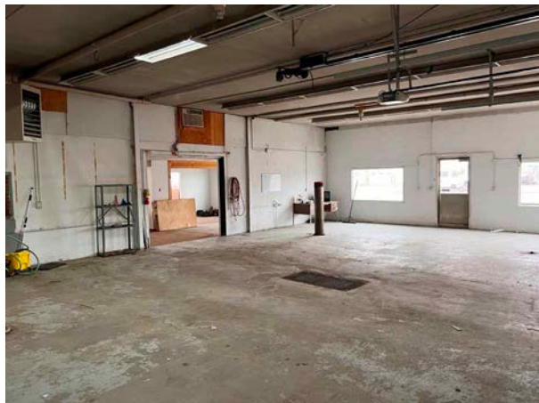
East Shop Space
