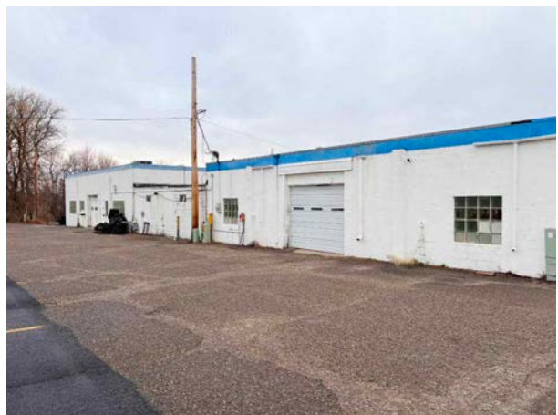
Subject Building - South Side
