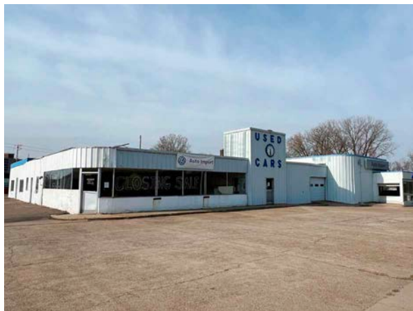
Subject Building - North Side
