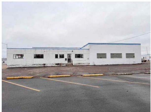
Subject Building - West Side
