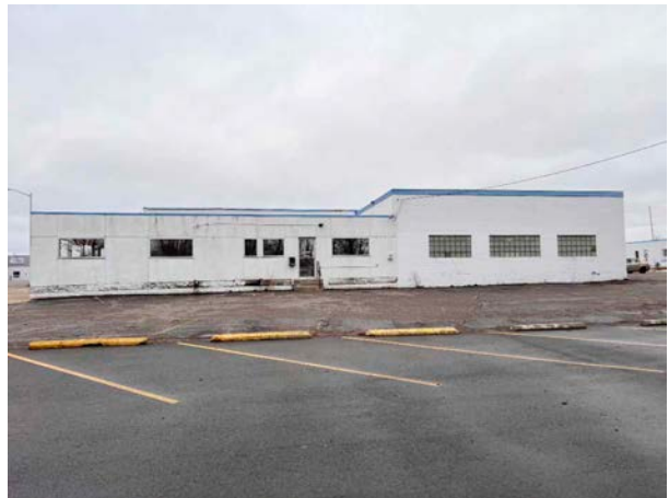
Subject Building - West Side
