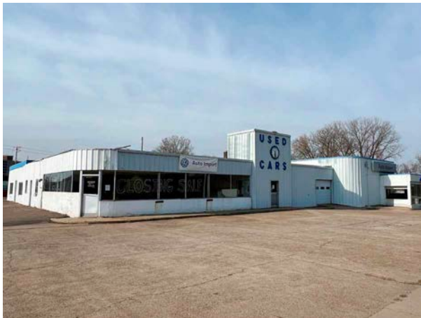
Subject Building - North Side
