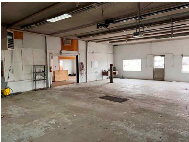
East Shop Space
