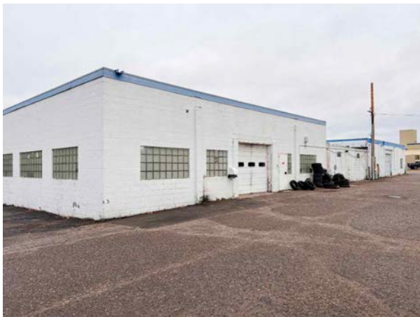
Subject Building - South Side
