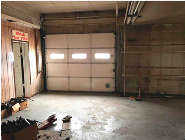
North Drive-In Door Area
