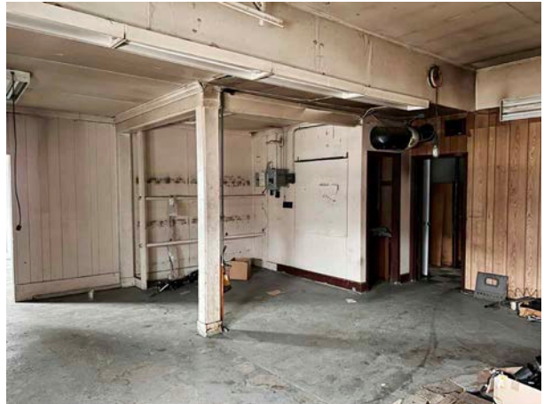
North Drive-In Door Area
