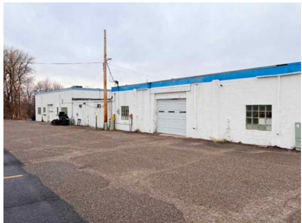
Subject Building - South Side
