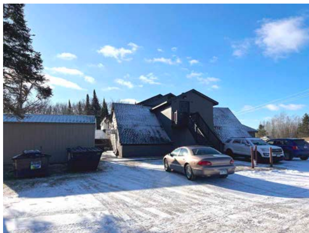
Upper Level Apartment Access & Smoke House
