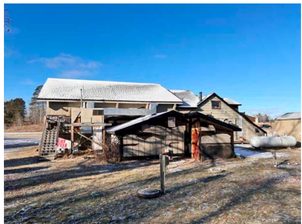
Back Side of Property
