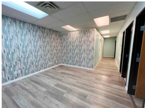
Bay 3 - Work Area
