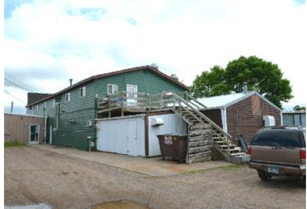
NW Side of Building
